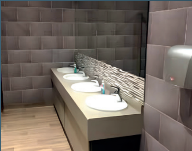
GREAT BROMLEY INSTALLATION
